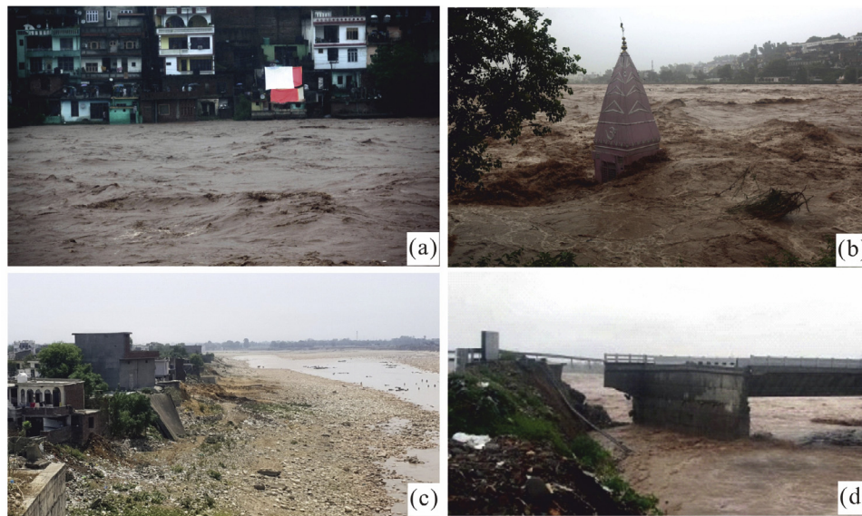
Fig. 10. (a-b) Havoc caused by flash flood in the Jammu city area, (c-d) damage caused by the flash flood in the river banks in Jammu city.
